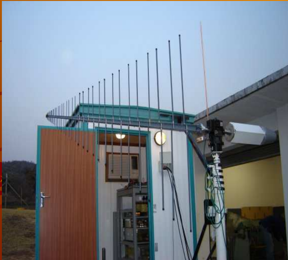
Complete antenna assembly
